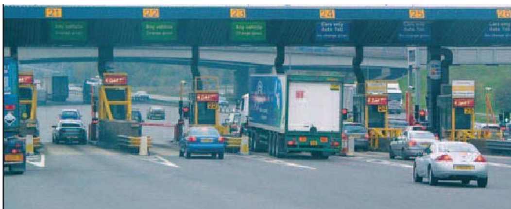
Figure 1 A toll plaza in the UK
