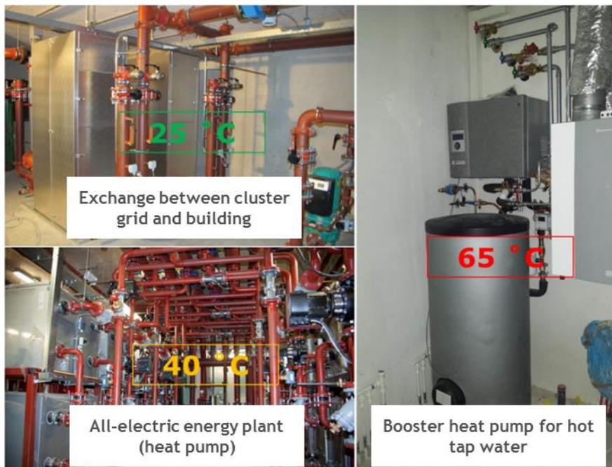
NB: The cited temperatures indicate the temperature level of the process shown.
