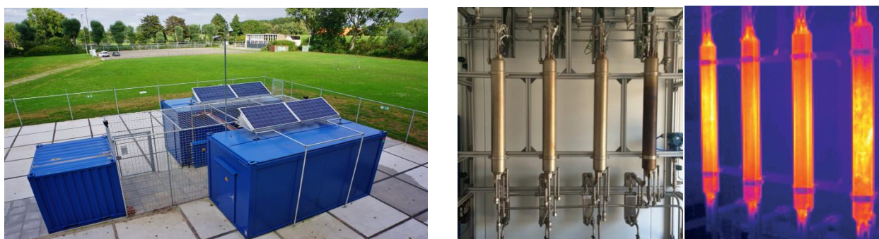
Figure 4-10 Power-to-Gas installation (left) and IR photos of the methanation process (right) of the Rozenburg power-to-methane project in the Netherlands, a project of Stedin, Ressort Wonen, Agentschap NL, Gemeente Rotterdam and DNV GL 32 .
