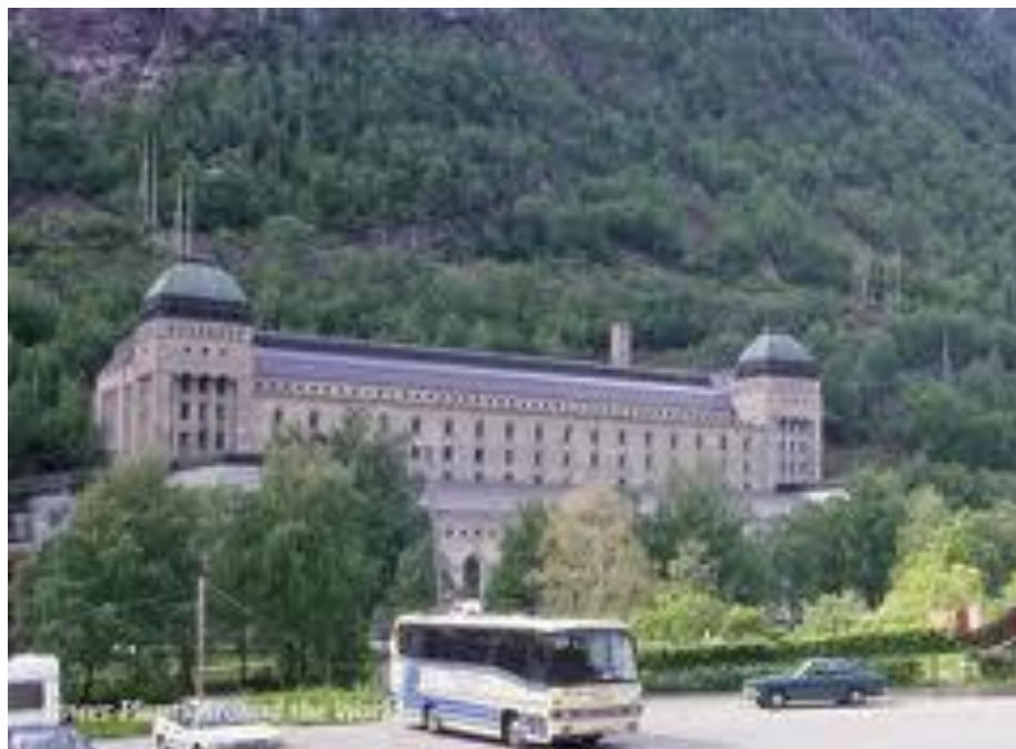
Figure 5 The Vemork power station at the Norsk H Rjukan reservoir
